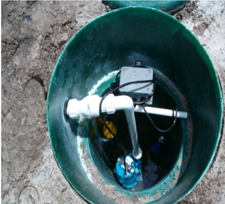
After the PEP Tank and control panel have been installed it is time for the installation of the pump assembly. The technician installs and terminates the pump as well as the plumbing necessary to complete the PEP System.
