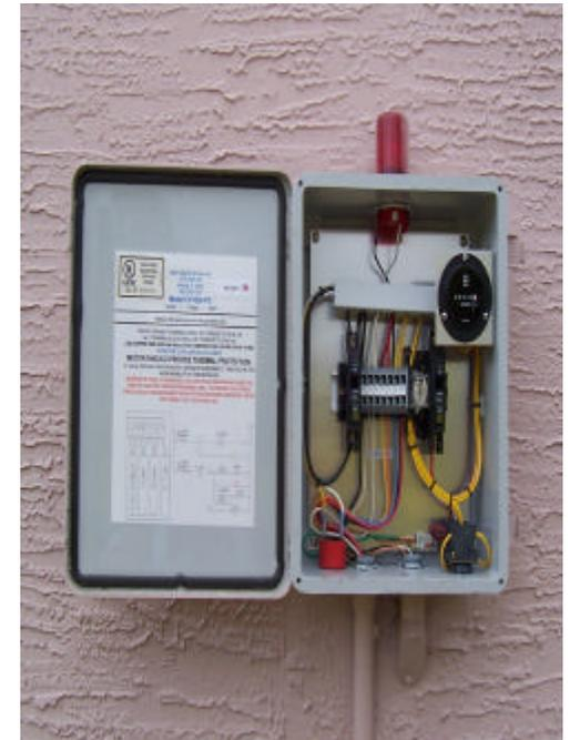
should always be illuminated. The red light is part of an audio-visual high water alarm. Should the PEP System malfunction, the red light will come on and an audible alarm will sound. If this happens, you should press the audible alarm button located on the bottom of the panel and call Customer Service immediately, **(386) 986-2360**.
