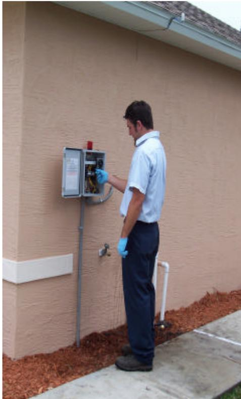
contracted licensed electrician. The panel houses all of the electrical components necessary to operate the system including the circuit breakers, audio and visual alarms and pump run clocks.
